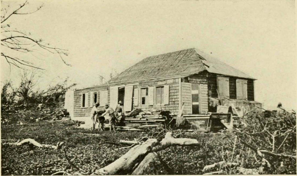
CANAAN ESTATE HOUSE, AFTER HURRICANE
