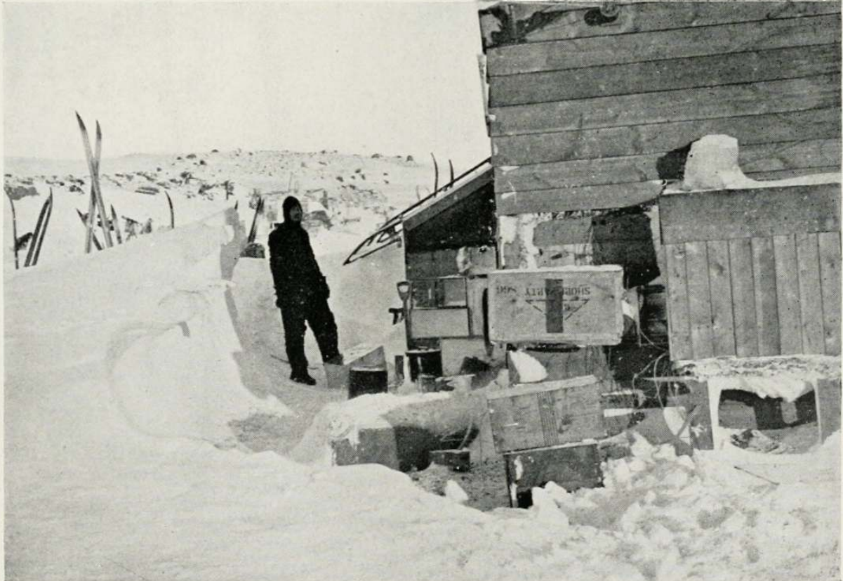
THE EAST CORNER OF THE HUT SHOWING THE EDDY TRENCH SCOOPED OUT BY BLIZZARDS ON THE WINDWARD SIDE OF THE HUT, SEPT. 14, 1911.
