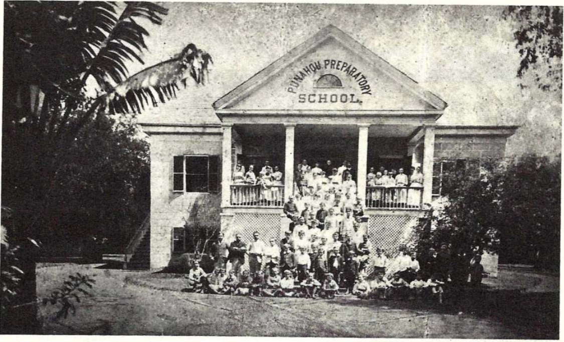
Punahou Preparatory School in remodeled Armstrong premises on Beretania. Presently a part of the site of St. Andrew's Cathedral.
