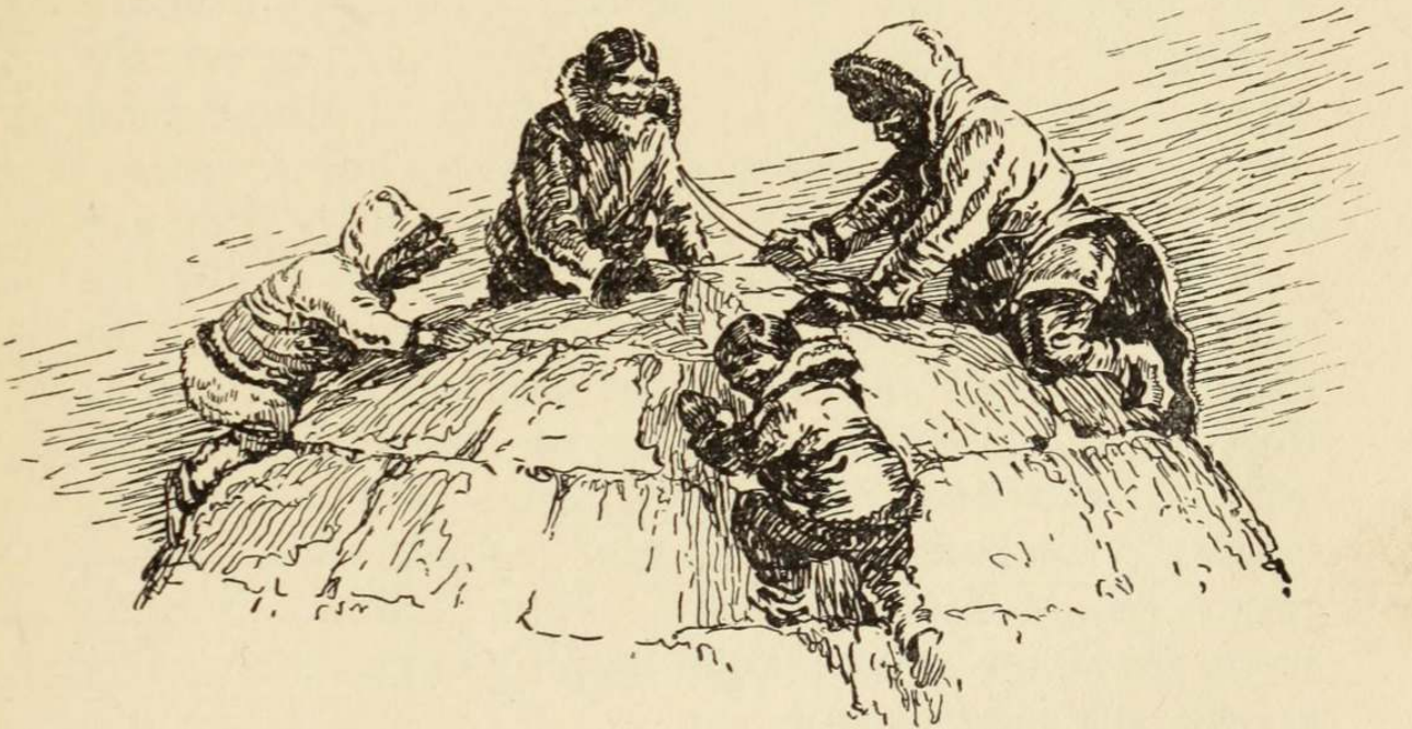
FAMILY ON ROOF OF IGLOO SHOWING STRENGTH OF CONSTRUCTION
