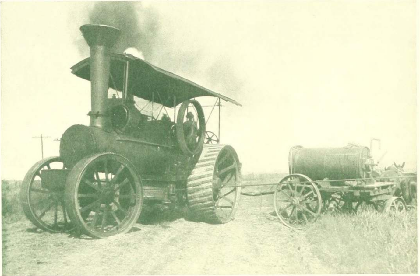
Steam Plow (taking on water) By means of a steel cable the plow or knifer is drawn back and forth
