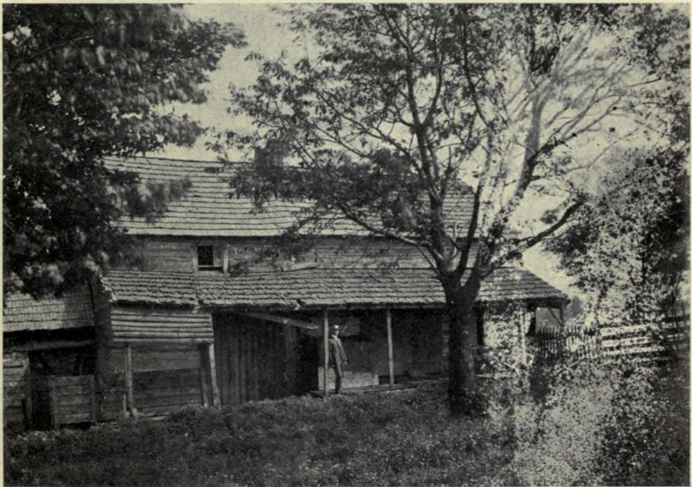
OLD FORT GADDIS, NEAR UNIONTOWN, PENNSYLVANIA
