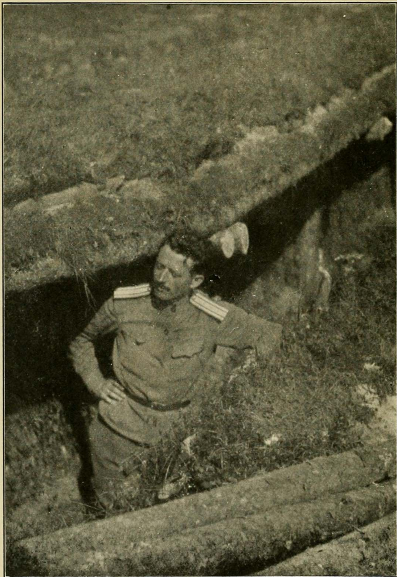
Surgeon Grow in a Russian trench. Note the trench's over-hang, built as a protection against shrapnel.
