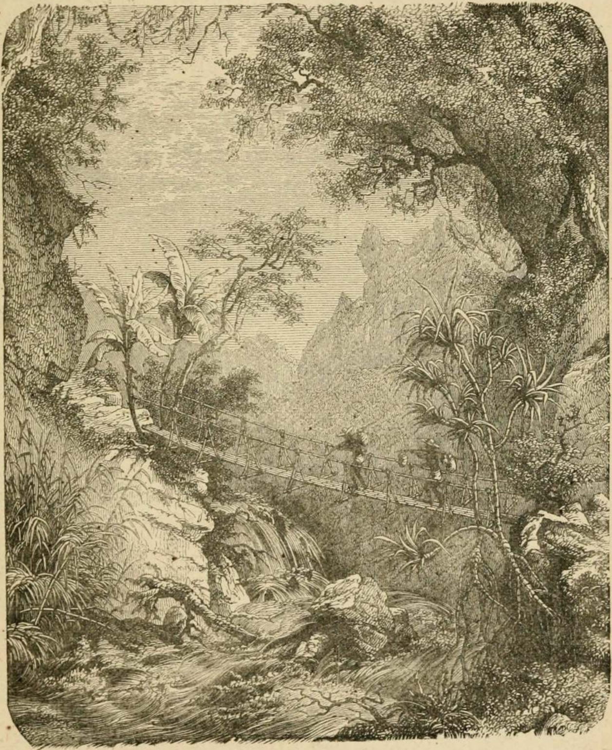
BRIDGE NEAR KABADI.
